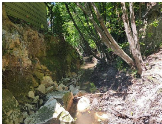
Significant bank erosion and private property loss
